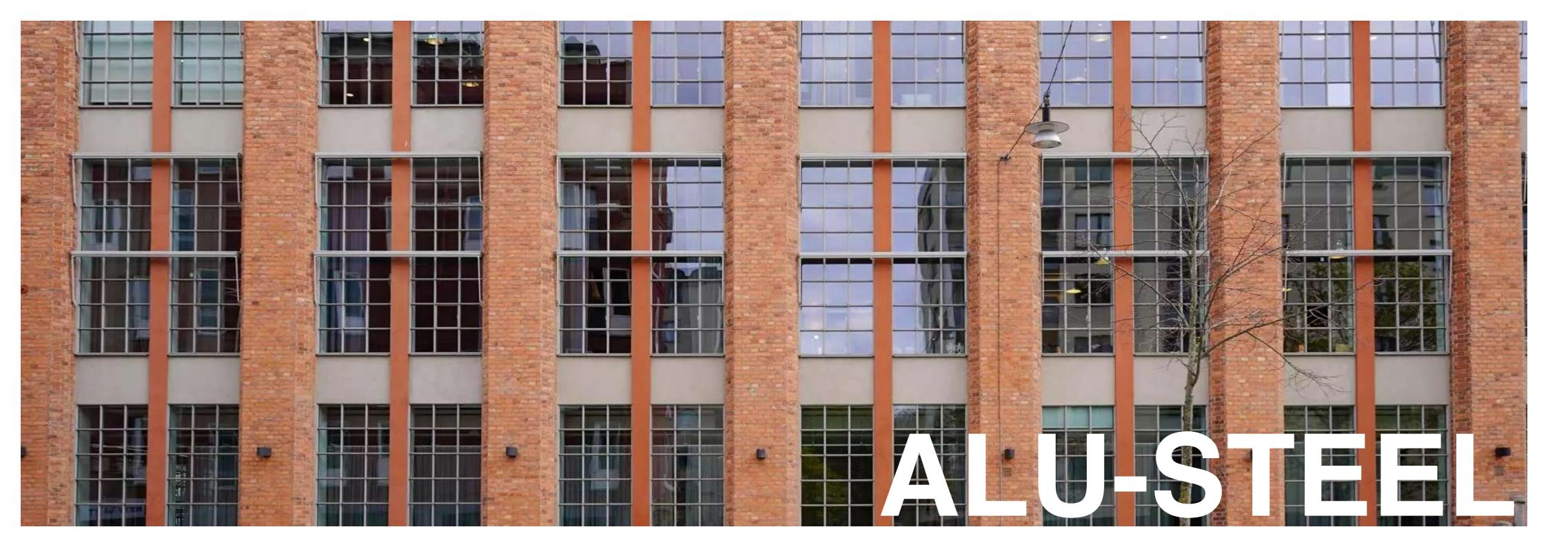
The ALU-STEEL line allows you to replicate the style of historic steel windows, but using extruded aluminium.
